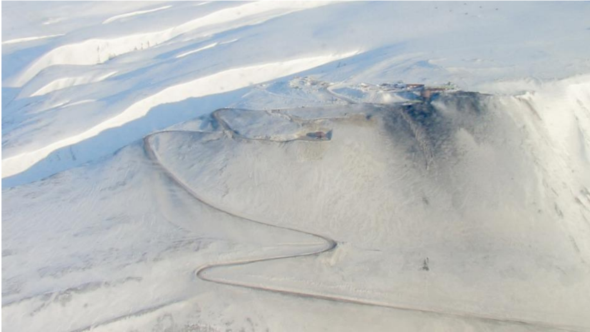
The road to Mine 7 outside Longyearbyen. (Photo: UNIS).
