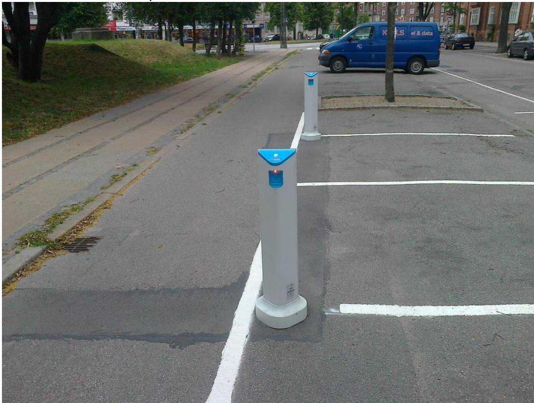
Figure 9: Better Place charging posts in Copenhagen summer 2013, shortly after the bankruptcy. Note the red light signaling out of service and the absence of electric cars. Photo: Mads Borup
